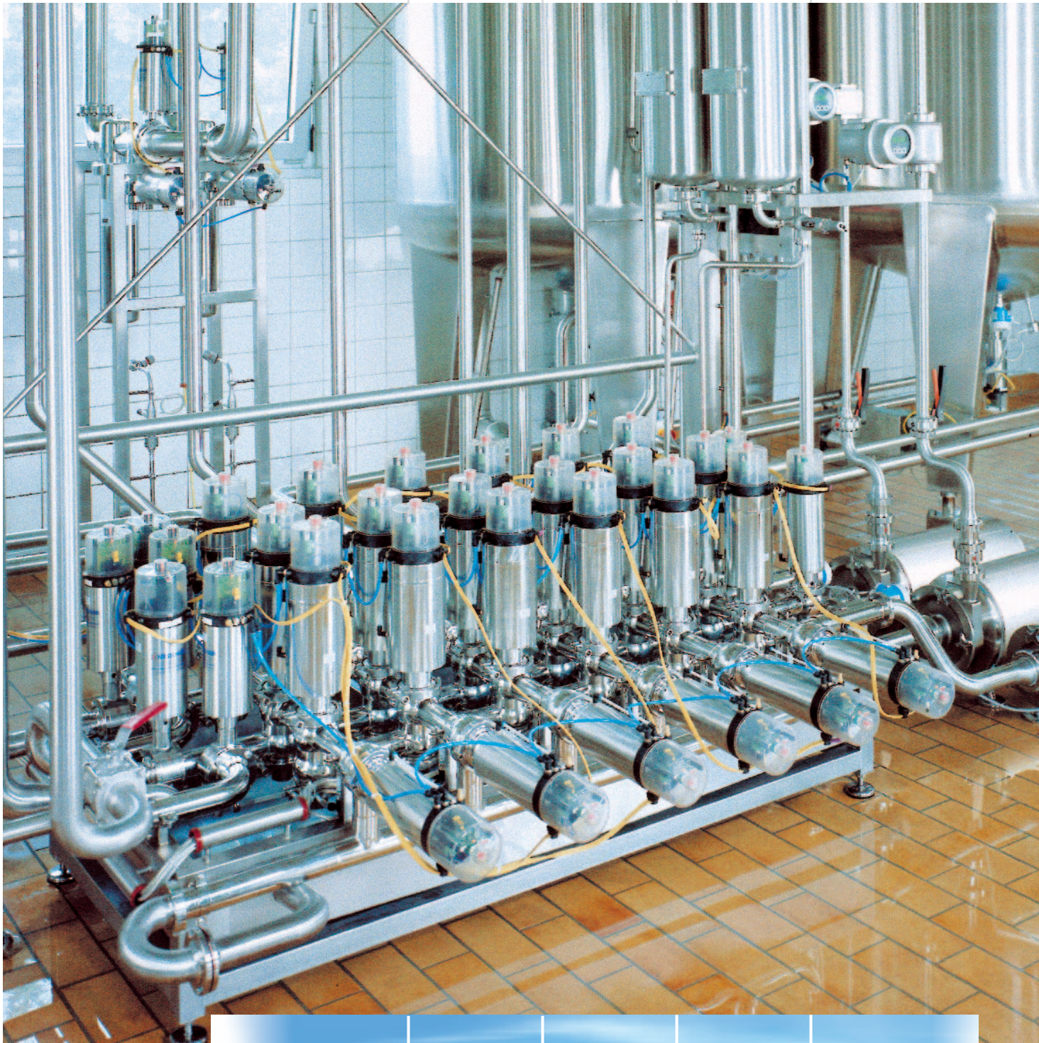
▲ Double seat manifold with ASI-Bus control system in a pharmaceutical production facility.
