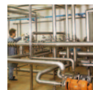
Particular test center for new developments and product control
